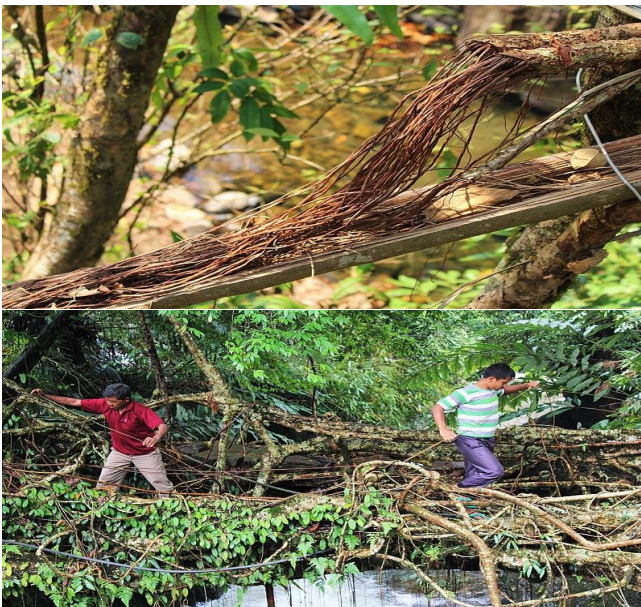
Fig.2. Living root bridge is formed by guiding the pliable roots of rubber fig trees
